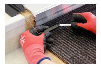
17. Fit the BLANK into the open end of the LR1238 TUBE.
