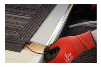
17. Cut to size and insert the DC1010 diffuser cover.
