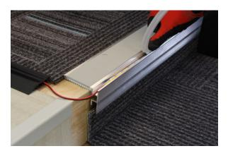
18. If the total LED Tape lengths exceed the stated maximum run, then the LEDs must be wired to the power supply as multiple shorter LED Tapes in parallel.
