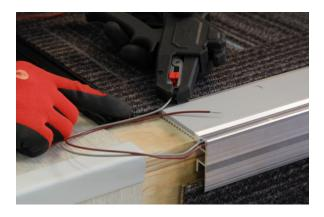
20. Crimp the wires using the correct size crimps.
