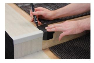
3. Measure between the back of the end cap that you have just marked on the front tread to the edge of the tread. This measurement determines the length of cable management required.
