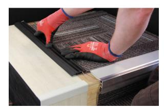
21. Install the end caps, inserting the lugs into the appropriate retainers.
