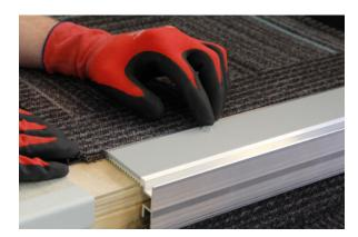
12. Place wiring into the appropriate cable management channel from the feed point.
