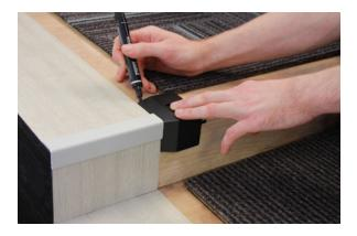
3. Measure between the back of the end cap that you have just marked on the tread to the front edge of the tread. This measurement determines the length of cable management required.
