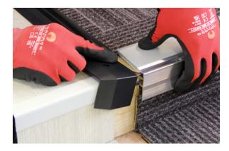
24. Secure the end cap with a screw and place the pip to cover the screw head.
