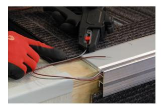
18. Crimp the wires using the correct size crimps.
